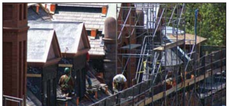
Close up of worker on the roof at 295 Huntington Ave.
